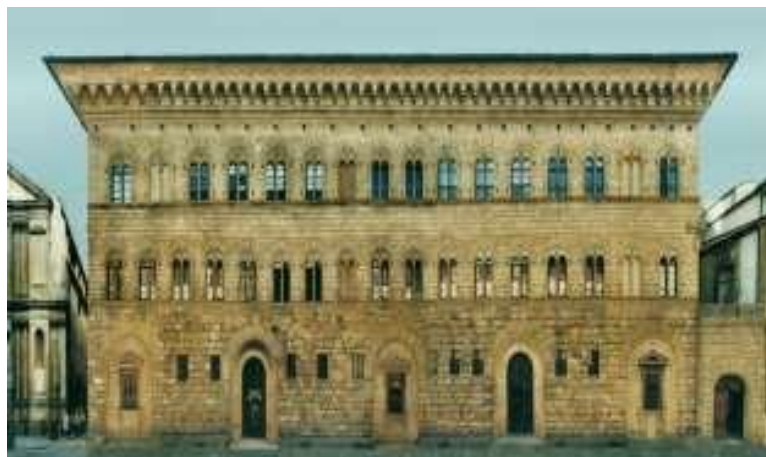
Figure 1. Palazzo Medici Exterior (Günel, 2016)
