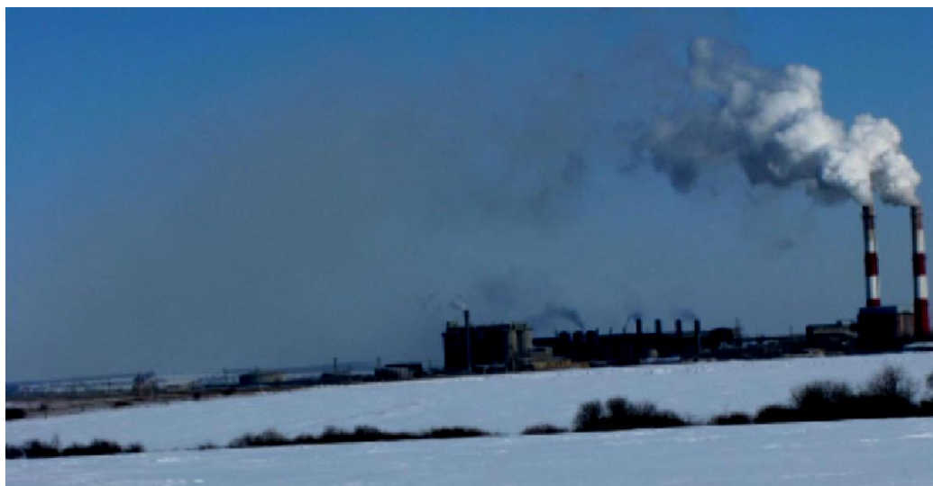
Figure 6. Mikhailovtsement CJSC: a descending stream of emissions with an anticyclone inversion and southwestern wind
