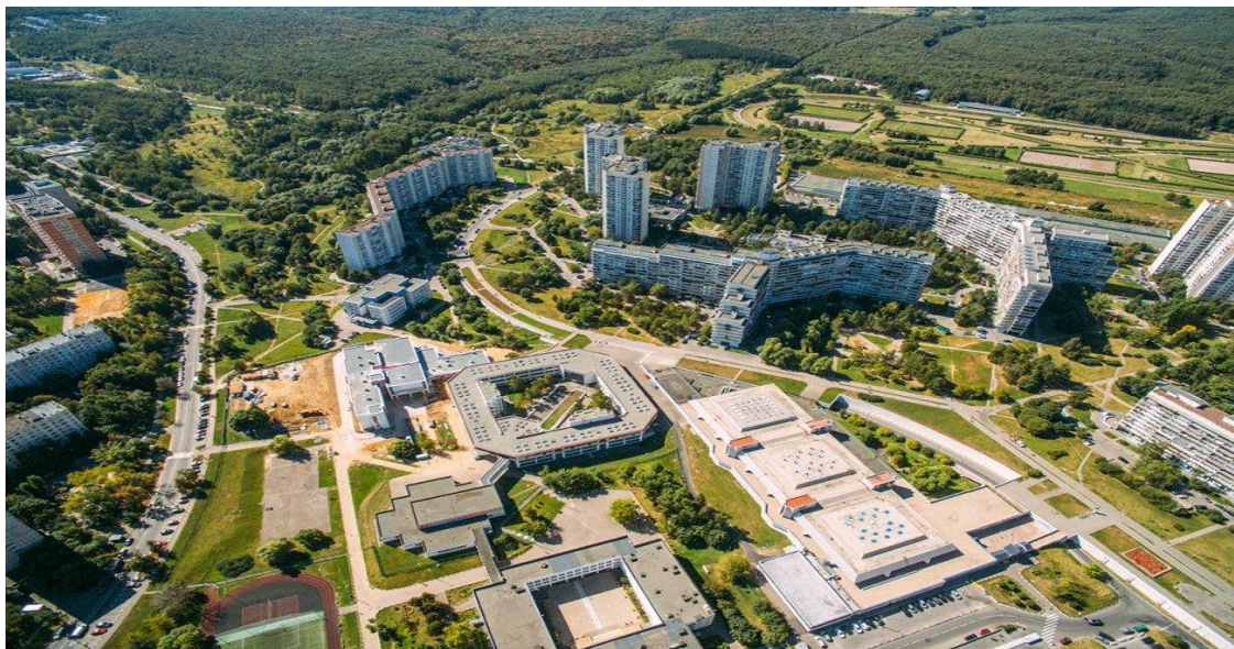
Figure 10. Example of the design of tunnel gallery over a city street and the creation of pedestrian boulevard on its upper covering (North Chertanovo, Moscow)
