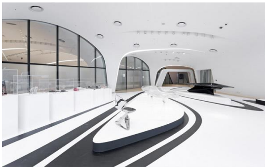
Fig.21. (a) GFRG ceiling material of Dongdaemun design plaza & park, (b) Aluminum cladding material of Dongdaemun design plaza & park
