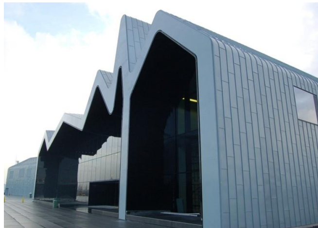
Fig.9. (a) GFRG ceiling material of Riverside museum, (b) Rheinzink cladding material of Riverside museum
