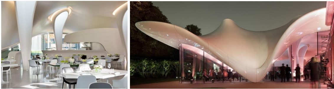
Fig.18. (a) FRP ceiling material of the curvilinear roof and columns, (b) GRP cladding material of the curvilinear roof
