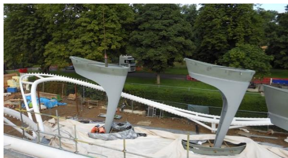
Fig.17. (a) Construction of shell structure system (DCS), (b) Construction of tapered steel columns
