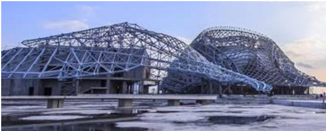
Fig.24. The space frame structure with RFC walls of Harbin Opera house
