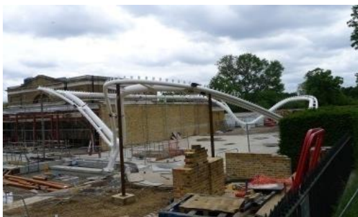
Fig.17. (a) Construction of shell structure system (DCS), (b) Construction of tapered steel columns
