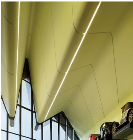
Fig.9. (a) GFRG ceiling material of Riverside museum, (b) Rheinzink cladding material of Riverside museum
