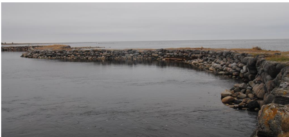
Fig. 1. Stone dam between Bolshoi Solovetsky Island and Bolshaya Muksalma Island
