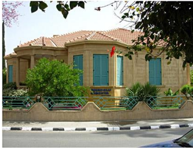
Figure 4- Elevation of The House Addressed Şerif Arzık Street No:38, Köşklüçiftlik / Nicosia (Author)
