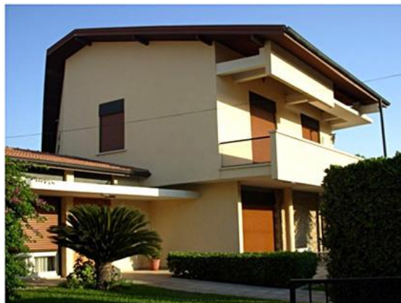
Figure 6- Elevation of The House Addressed Server Somuncuoğlu Street No:4, Köşklüçiftlik / Nicosia (Author)
