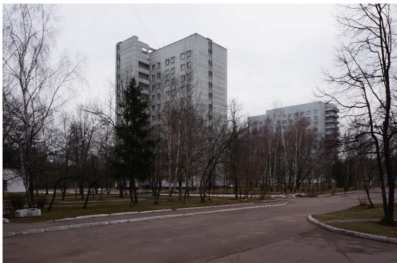
Figure 2. The campus of Moscow State University of Civil Engineering in Moscow. Functional potential of the complex is not revealed.
