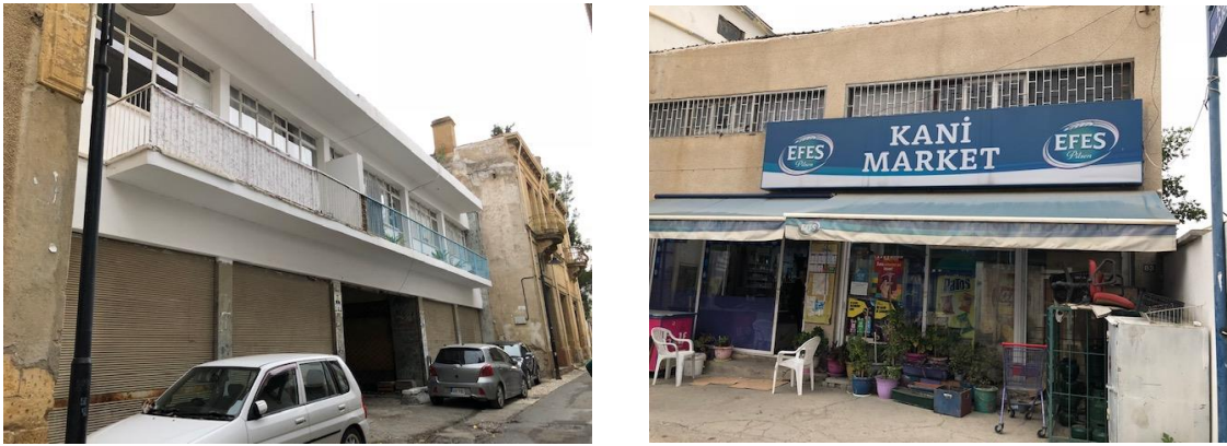
Figure 13. a, b. Frame Structure System Buildings in Victoria Street (Author - 2020)
